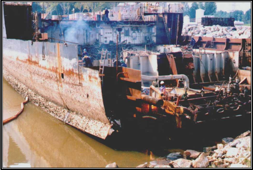
USS Plymouth Rock being dismantled
